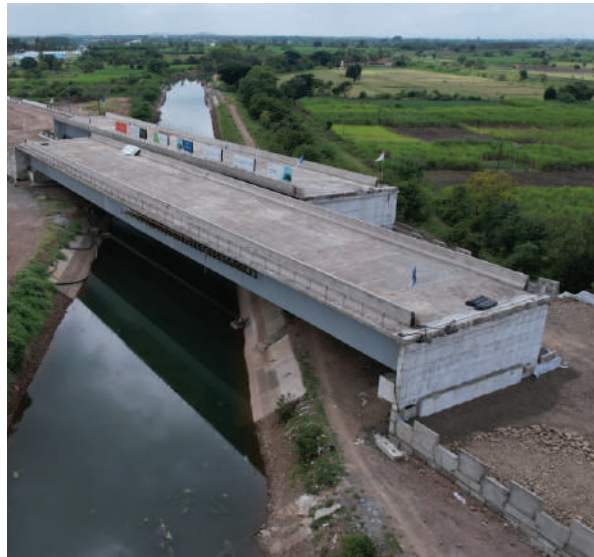
102.6-meter Single Span Bridge (UHPFRC) (Shot at location)
