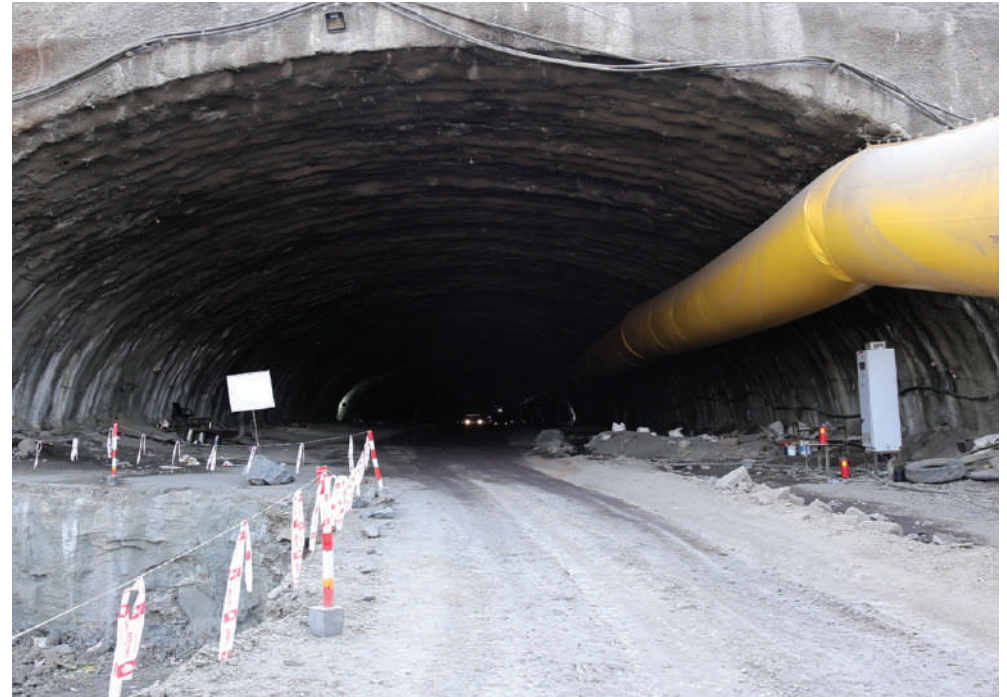
Long Twin Tube 8-Lane Tunnel, Mumbai (Shot at location)
